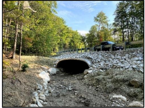
Clover Mill Road Stream Crossing
