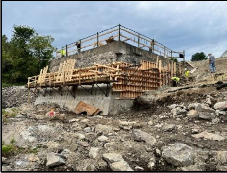
Historic Overlook Stabilization
