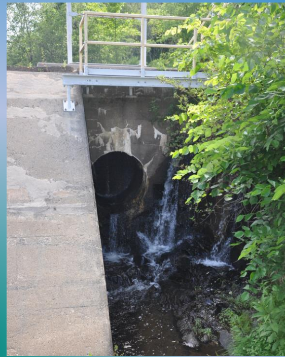
3' diameter orifice sluice gate
